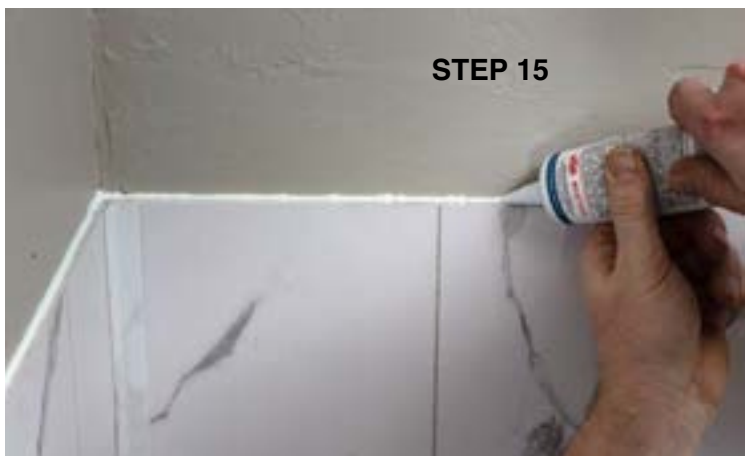
Apply sealant to top edges of all the panels for a watertight seal.
