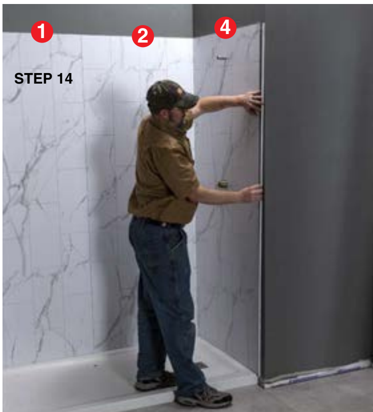
Install the J-trim to cover the outside edge of panel 4.
